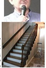
he stained to match other woodwork in his house. Chuck made the risers of poplar. Each tread was custom cut to fit thus avoiding the generic cut board and tons of caulk which he said a contractor would do. Certainly a step in the right direction.
