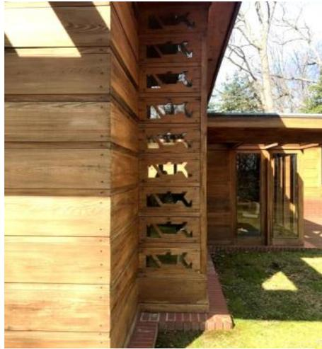
Exterior of home showing small windows with cutouts. The exterior was recently cleaned and treated with a protective coating (not stained).
